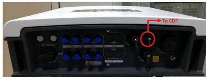
Figure 1: Connection between a CDP and single inverter.
