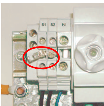
Fig. 5-5 .- Jumper for short-circuiting the secondary winding of the current transformer (TC).
