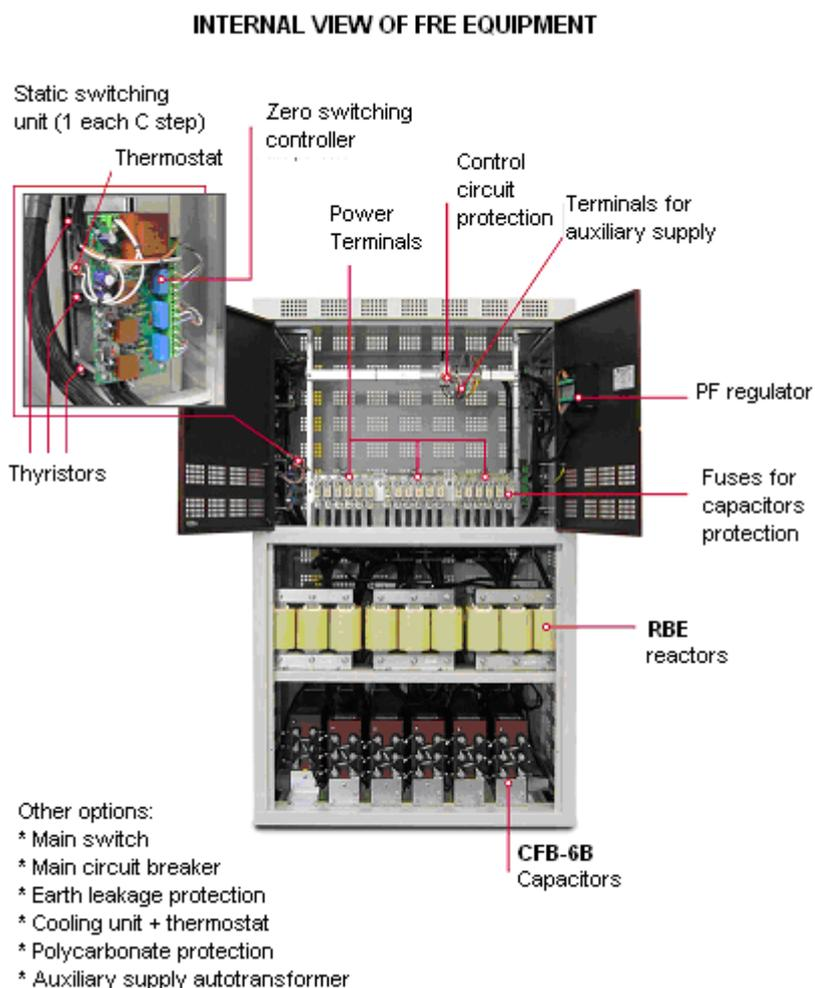
Fig. 4-3 .- FRE Capacitor bank components
