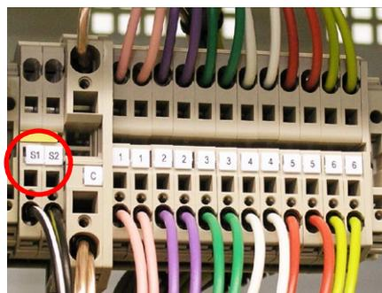
Fig. 5-3 .- CT connection terminals
