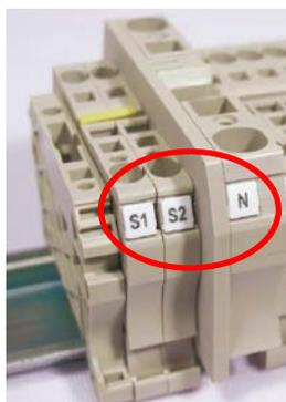
Fig. 5-4.- CT and neutral connection terminals if required
